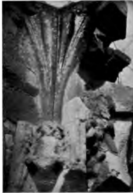
St. C. B. N.E. ANGLE OF CLOISTER SHOWING INSERTED CORBEL OF XV. C.
